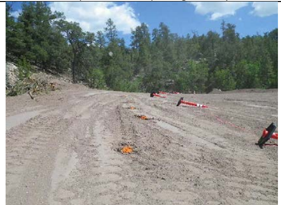
Soil sample areas. High winds blew the delineators down.
